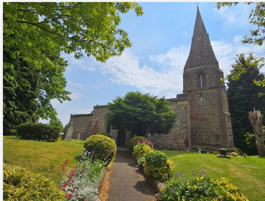
Figure 15: St Michael's Church, Diseworth– Grade II* Listed
